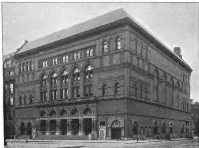
CARNEGIE MUSIC HALL, SEVENTH AVENUE, SOUTHEAST CORNER OF 57TH STREET.
